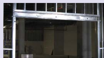
A lintel system used in a loading dock, where there is a large amount of lined wall area above the door opening.
