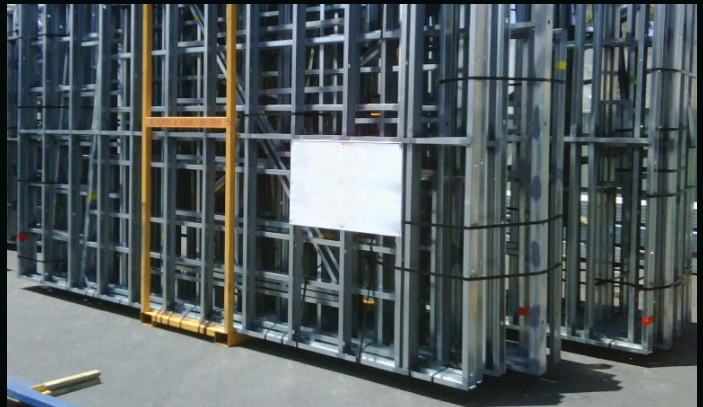
Steel framed housing modules waiting to be transported to the Outback, for use in affordable housing for Australia's indigenous communities.
